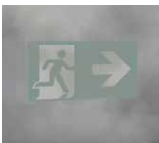
Badly illuminated escape sign
